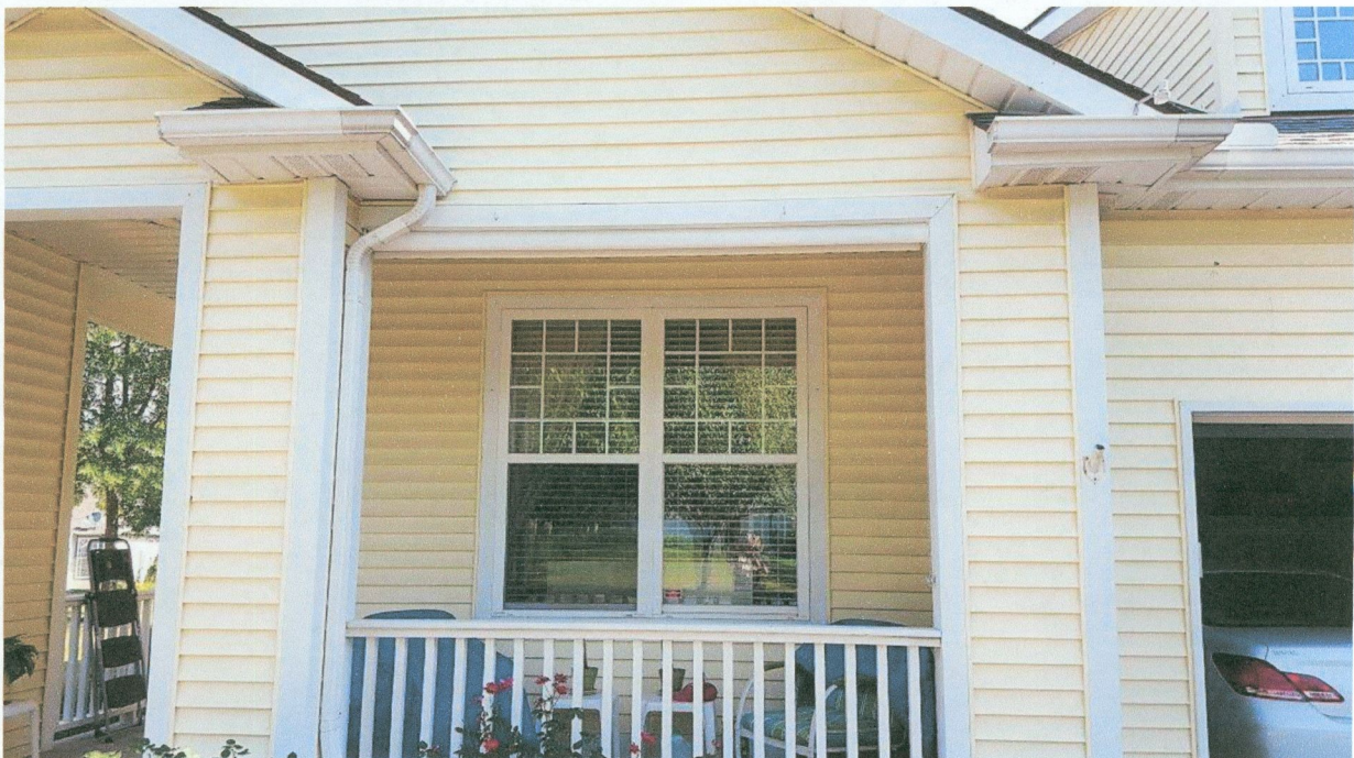
Solar shade in closed position
