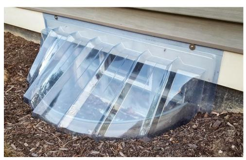
This well is screwed into the flashing so if the covers are damaged or old and need to be replaced with a flat type, or are not being replaced, it is the responsibility of homeowner to seal with silicone.
